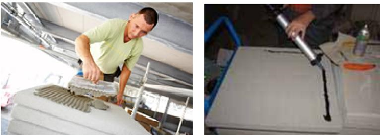
Use only low shrinkage adhesive PCI Nanolight to maintain fire rating,
