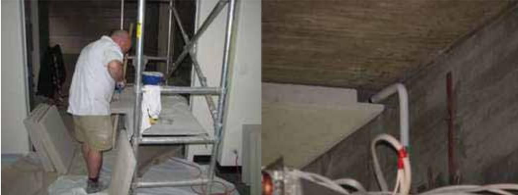
Pictures show hand cutting with handsaw. Next picture shows back of panel routed out to allow for conduit to be hidden.
